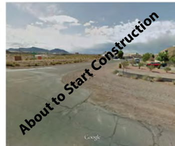
Appaloosa Storm Drain Project
