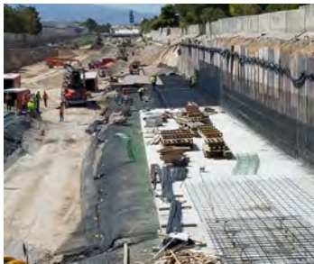
Las Vegas Wash- Sloan Channel to Stewart Ave and Flamingo Wash
