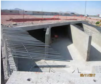
Pittman North Detention Basin and Outfall Phase II- Starr Avenue
