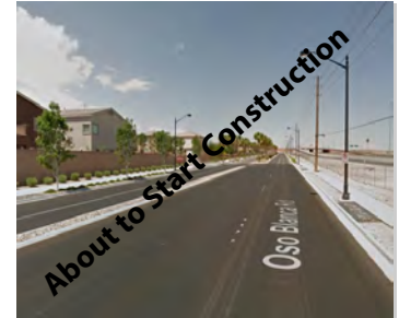
Central Freeway Channel at Cheyenne
